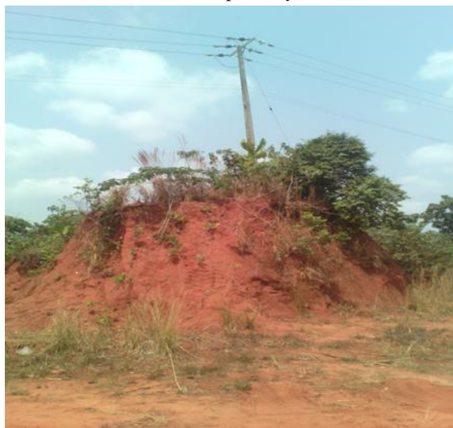
Plate 4: Showing an affected electricity Pole in the area at the point of collapse
